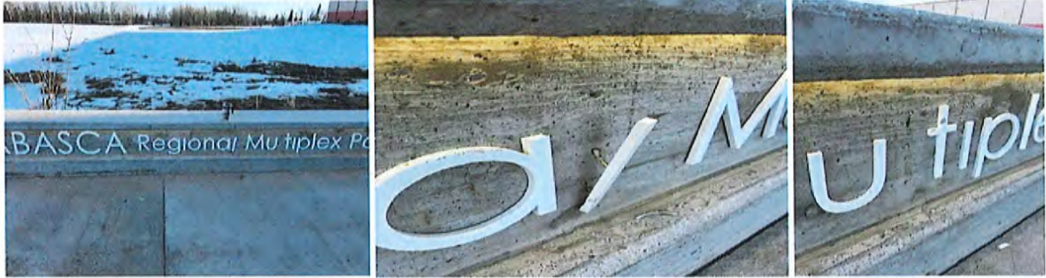
West side pool sidewalk
